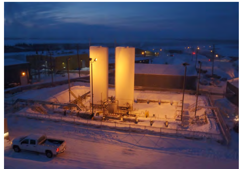
Figure 23 NTPC's Inuvik LNG Storage Facility
